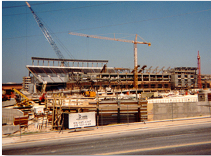
Darrel K. Royal Memorial Stadium Renovations, Austin, Texas
