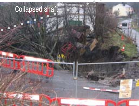
Subsidence damage
